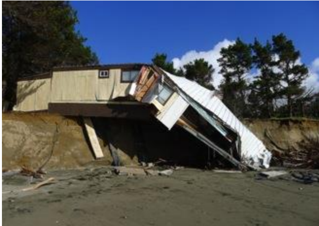
Bluff erosion destroys a house on Washaway Beach.
